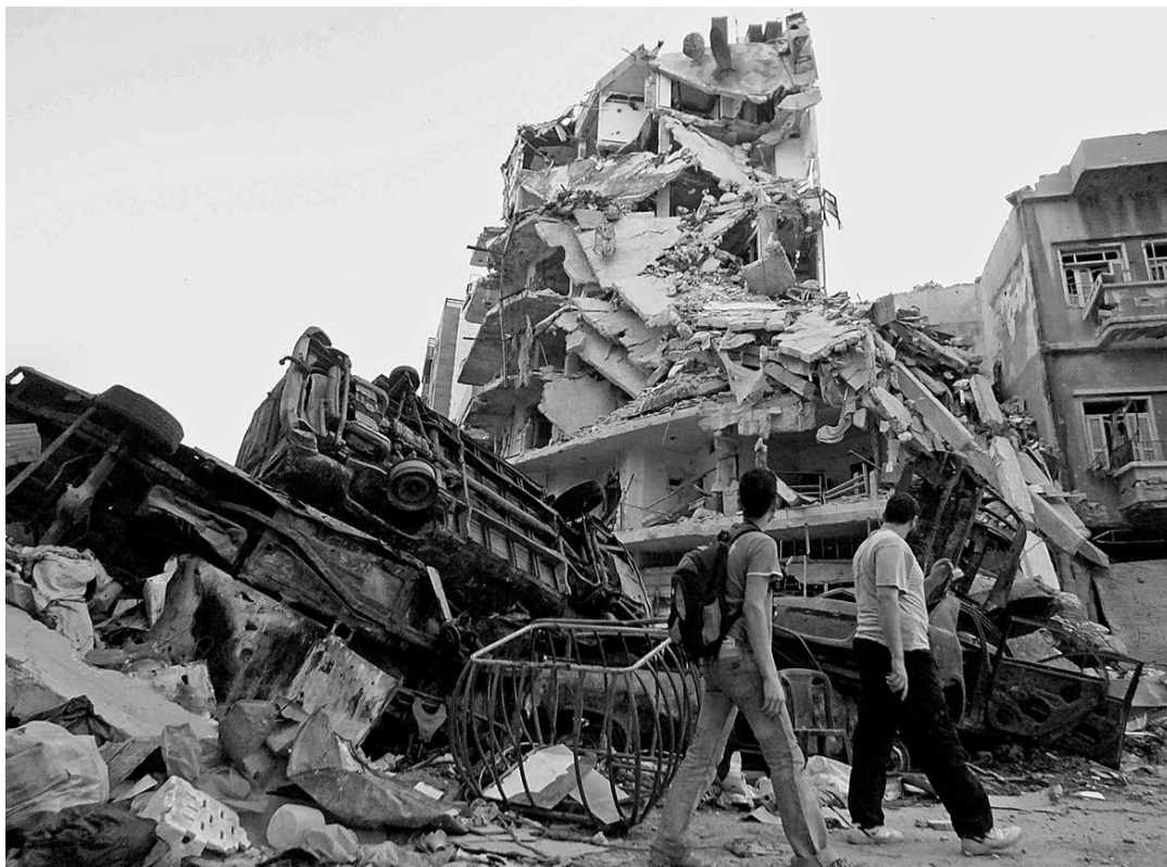
Damaged buildings in the Syrian city of Homs, where, humanitarian groups say, the fighting has become so fierce that many civilians are trapped and efforts to send in aid have been thwarted.
